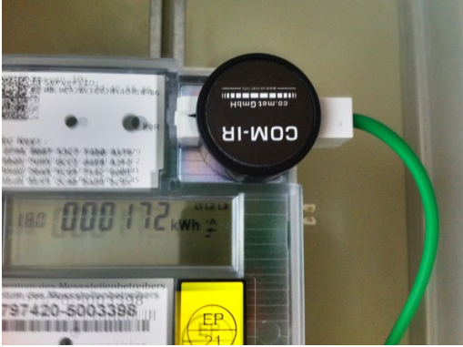
Figure 2.4: Optical sensor that reads fine-grained consumption data from a smart meter through an infrared interface. [214]
